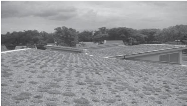
Extensive green roofs employ succulent low-growing plant species, such as sedums.
