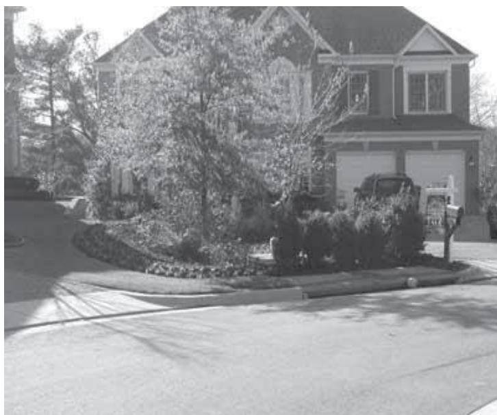
Bioretention facilities intercept stormwater runoff and use plants and soil layers to remove pollutants.
