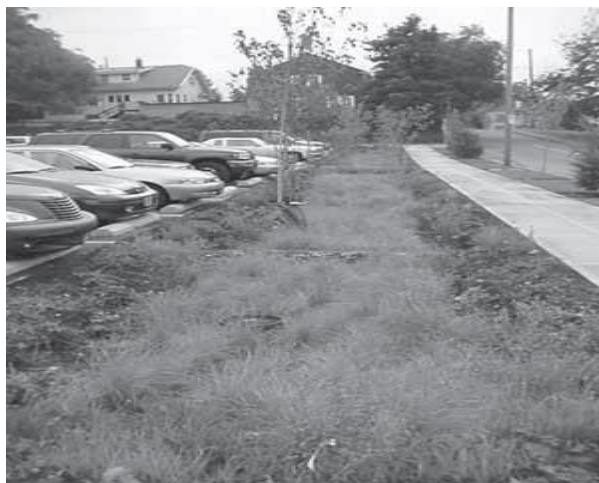
Vegetated swales are often located along roadways, parking lots and other impervious areas
