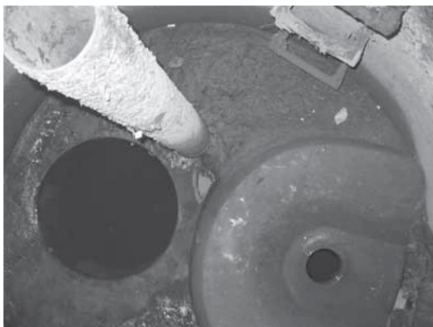
STORMCEPTOR-Manufactured BMP's are used solely for water quality enhancement in areas where space for BMP's is not available.
